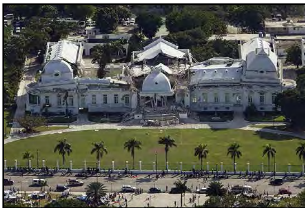
Haiti's Presidential Palace was badly damaged in the earthquake. The building was considered by some as a symbol of excess in a desperately poor country.
